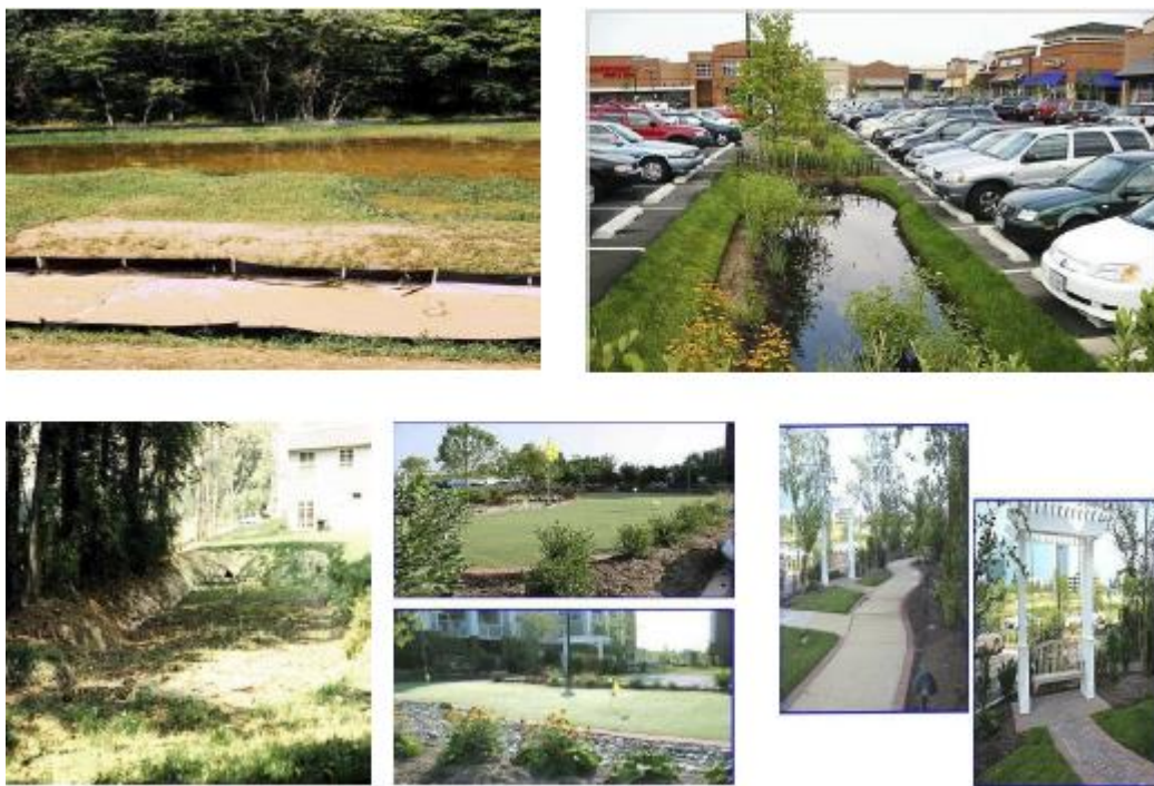
Figure 7. Numerous innovative quality pretreatment practices – sand filter discharging to a wetland buffer area, parking lot bioretention, stream-side pocket vegetative filtration area, pervious golf green and pathways.
