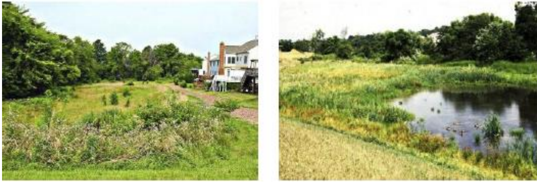
Figure 4. Newly created vegetative filtration buffer and habitat for nonpoint source flow management
