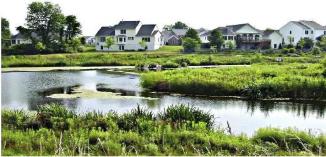
Figure 5. Constructed “horse shoe” pond for combined water quantity (flood) and quality management with pre-treatment and wetland habitat for additional resource and water quality benefits.
