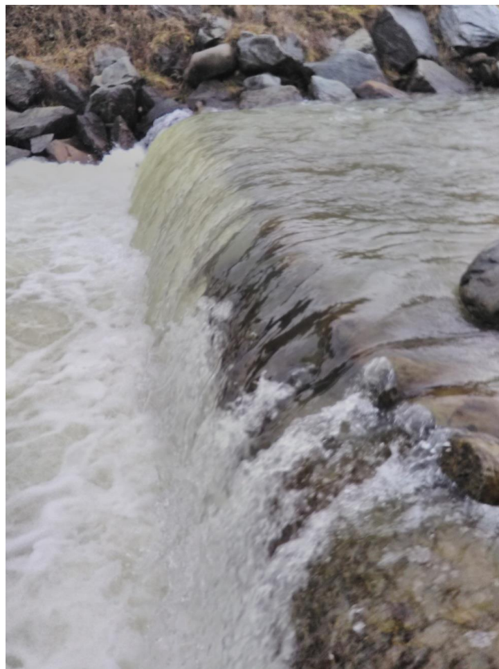
Figure 1b The discharge sill made from a tree
