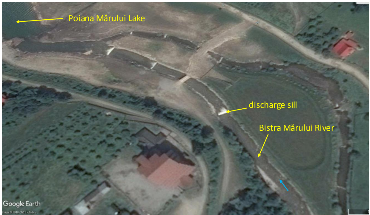
Figure 1a. Discharge sill located on the Bistra Mărului River (google earth.com)
