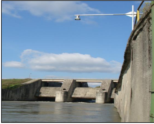
Figure 2. Installation with radar sensor
