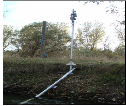
Figure 3. Installation with water pressure sensor
