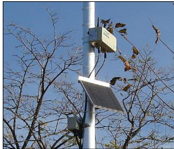
Figure 4. Adcon A753 GPRS RTU and solar panel.
