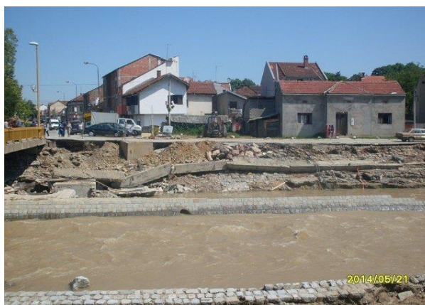
Figure 2. Damage caused to the left bank of the river Kolubara's regulated bed Source: Malesevic Dj., Valjevo
