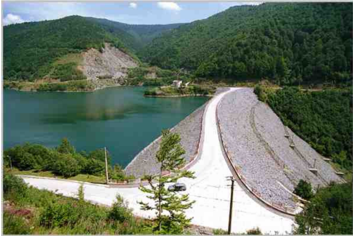
The Râușor dam on Râul Targului at the confluence with Zănoaga River
