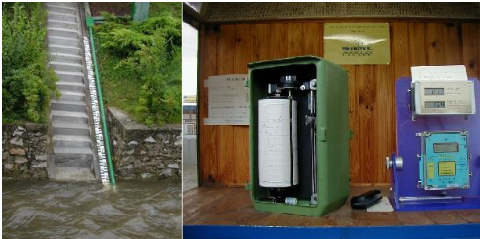
Figure 1. Hydrometric station and automated stream gauge device (SHMI)
