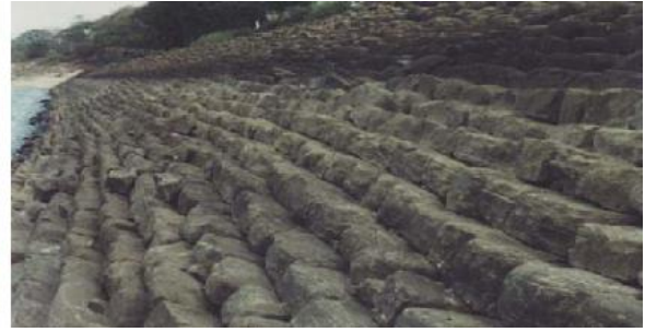
Figure 10. The stone placement in the Giritale Dam in Sri Lanka, built in the period A.D. 608-618 (after www.icold-cigb.org , 2013)
