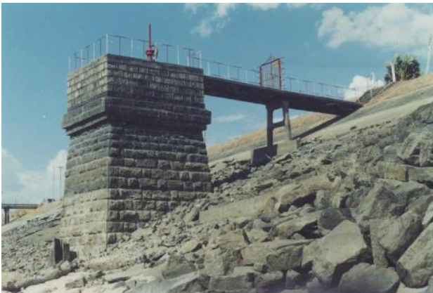
Figure 11. The ancient Minneriya tower built in the period A.D. 276 -303 in Sri Lanka. It was restored in 1901 and it is destined to irrigations (after www.icold-cigb.org , 2013)
