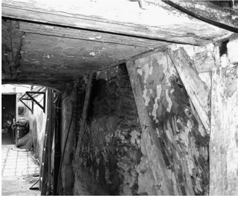
Figure 4. Photography documenting the condition of the half-timbered building before refurbishment
