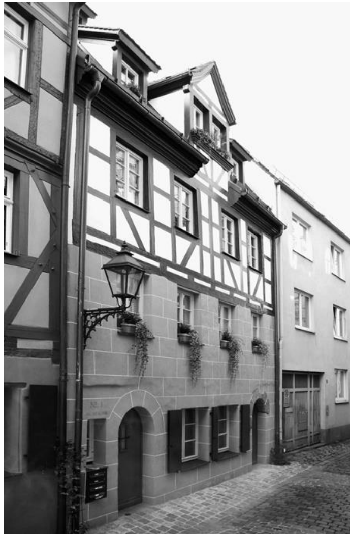
Figure 5. Exterior view of the timber-frame construction after renovation (photos by Alexandra Fritsch)
