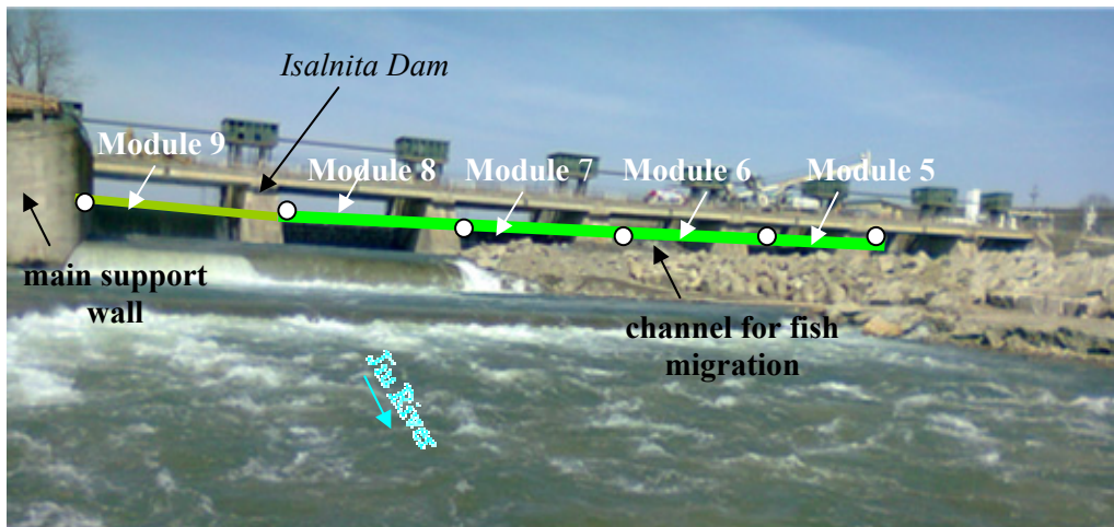
Figure 5. Positioning of modules 5-8 on the support pillars of Isalnita Dam - indicative scheme
