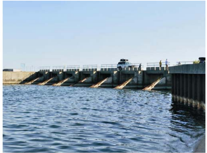
Figure 6 - The dam separating North Aral Sea from South Aral Sea (in the area of former Kokaral island), which allowed the rehabilitation of North Aral Sea (Photo by Vadim Bondar)
