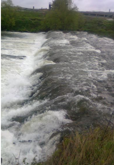
Figure 7 Discharge sill (bottom sill) in Apahida
