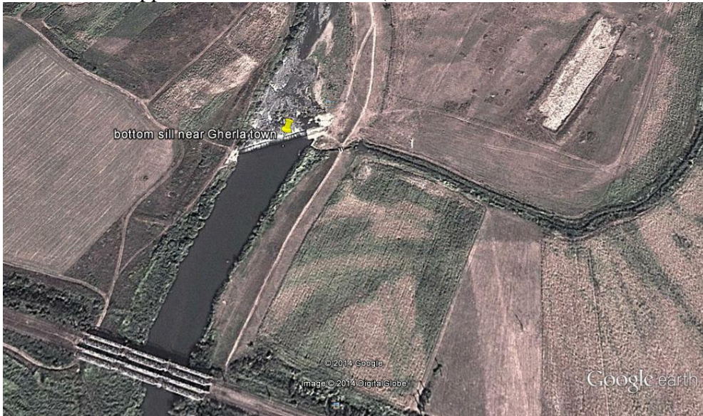
Figure 1 Bottom sill near Gherla town (Source: Google Earth, 2014)
