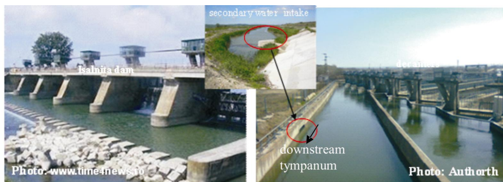
Figure 2. The Ișalnița water intake with the diversion dam
