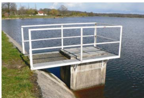
Photo 2: Monk cage in the form of an enclosure at Chaume Pond (commune of Azérables) seen from the dike (photo L. Touchart, 2008)
