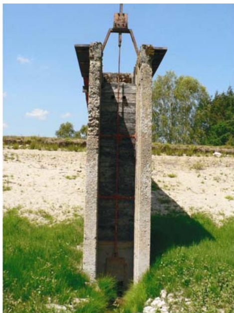
Photo 1: Monk cage with three walls at Ribières Pond (commune of Monteil-au-Vicomte) seen from inside the body of water while dry (photo L. Touchart, 2006)
